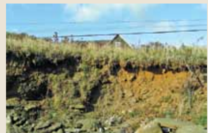
Erosion damage on a seaside road.
