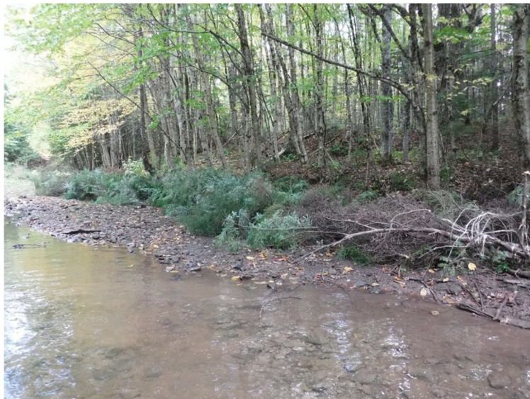
Figure 4 Showing completed brush mattress located on inside bend of meander, viewing downstream.
