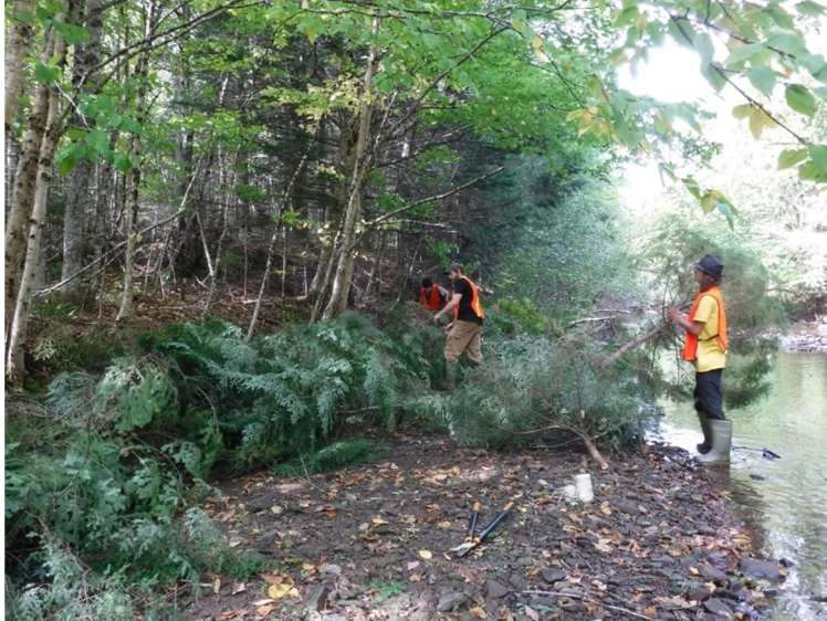
Figure 3 showing SAA field staff installing the brush mattress, viewing upstream.
