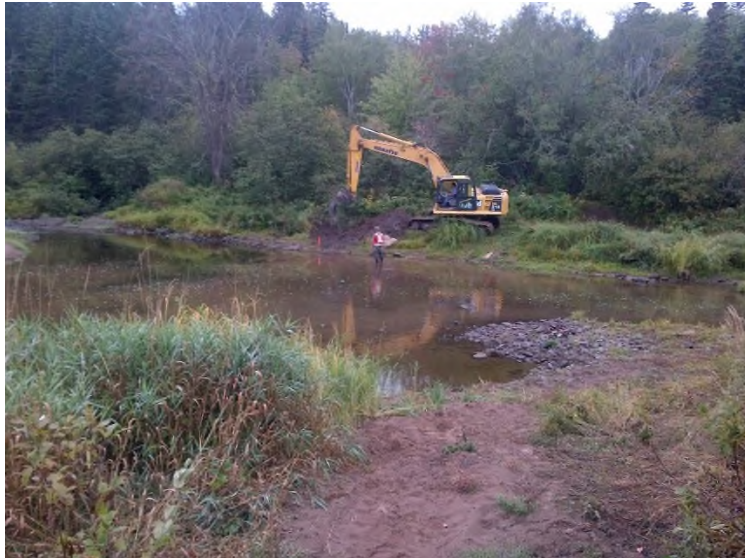
Construction of Rock Spur (Deflector)
