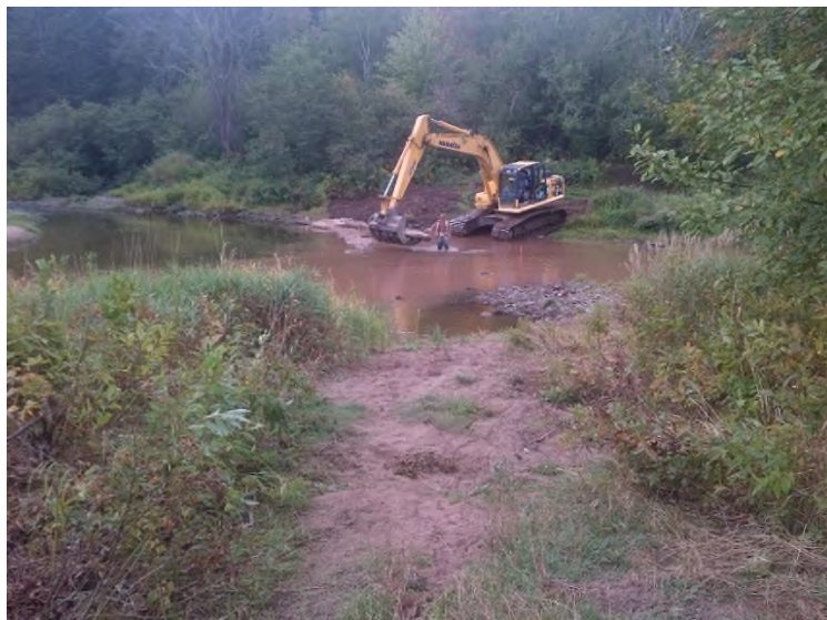
Construction of Rock Spur (Deflector)
